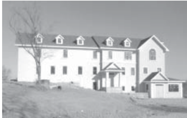
The new Regina Coeli House, shown after the windows and exterior doors were installed.
